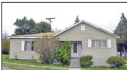
WEED . 1700 square foot, 3 bedroom, 2 bath home with loads of potential and a gorgeous view of Mt. Shasta. Located across Hwy 97 from Lincoln Park. #102115 Only... $44,900.
