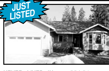
NEVER LIVED IN - 3BD/2BA 2096sq.ft. custom home. Nice front porch&back porch. Lots of tile counter space/cabinets in kitchen. Forced air cooling, oil/elect. heating. Large walk in master closet. $329,000 #97419
