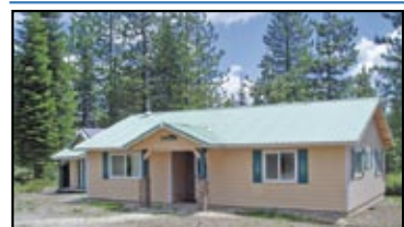
NEWER CABIN IN THE WOODS. Corner 2.5 acre parcel with Mt Shasta view. USFS land across the road. Well is 120'; produces 20gpm. DC pump, solar, storage tank and controller. Generator, installed 2 KW solar power for house. Maple cabinets, vaulted ceiling great room. Washer Dryer dishwasher all plumbed in. Shed & wood storage area. #100907 $205,000.
